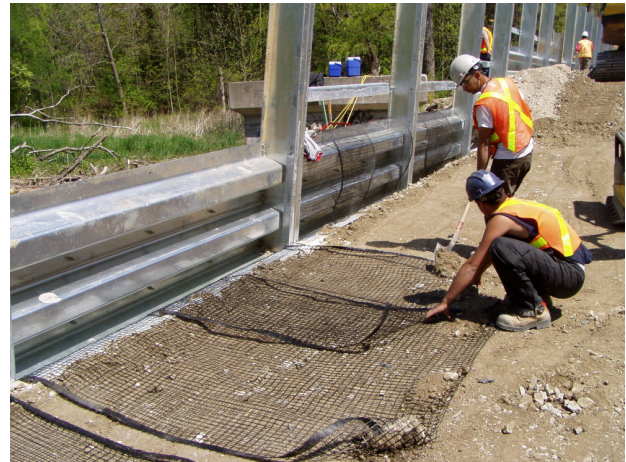
Figure 5 Wrapped connection for geogrid reinforcement
