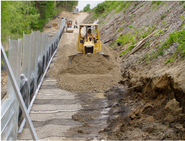
Figure 6 Backfilling operation over geogrid
