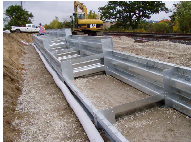
Figure 2 One of the true Bin-Walls during assembly
