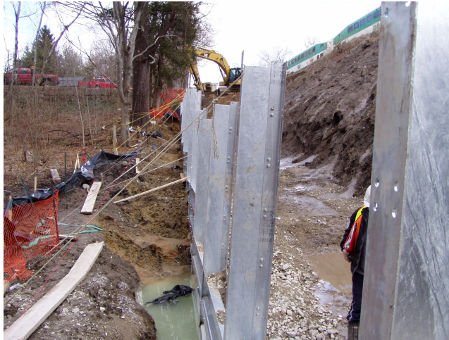
Figure 3 Non-typical bracing of wall fascia
