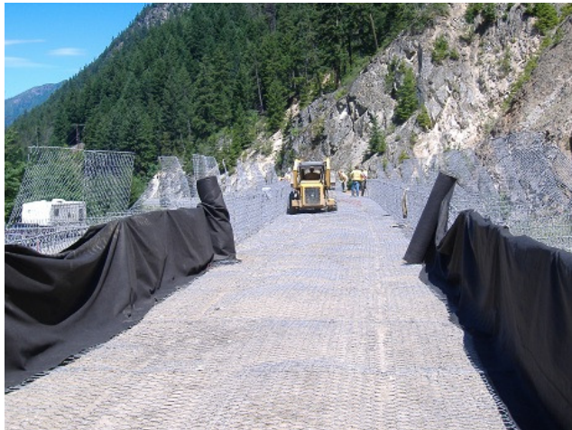
Figure 5. Reinforced soil units prior to placing structural backfill. Looking north.
