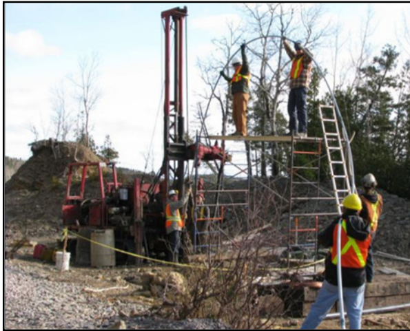
Figure 5. Vertical installation of SAA already inside PVC conduit.
