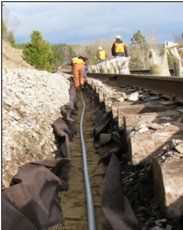
Figure 6. Horizontal installation of MEMS array inside PVC conduit in a trench in the rail bed.
