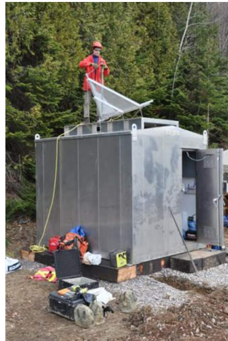
Figure 6. Photo of corner reflector CR2 installed on the roof of a utility bunker at the Gascons site.
