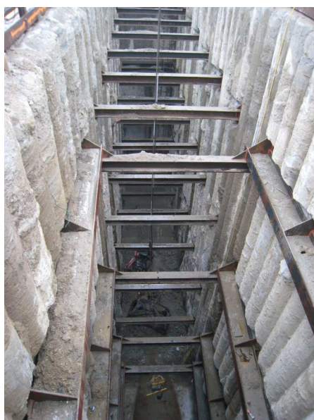
Photograph 1. Recovery shaft
