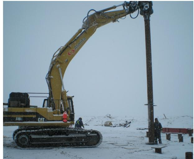
Figure 2. Typical helical pile installation
