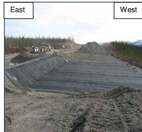
Figure 7: Placement of the heat drain across the full width of the embankment (section 2)
