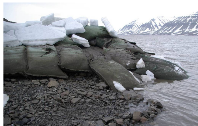
Figure 15. Visual inspection in 2009. Contact of the ice on the west corner One hole on bag 26, second on the left.
