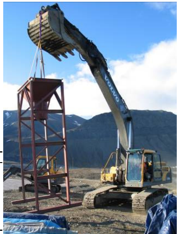
Figure 6. Elevated funnel used to fill the bags on site.
