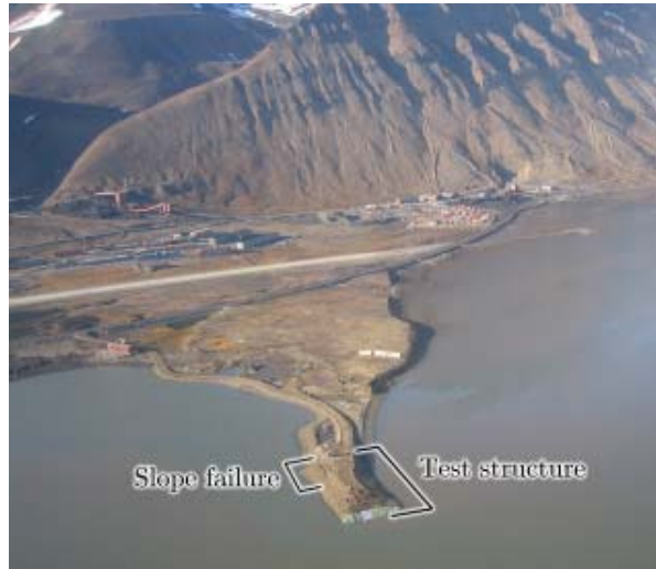
Figure 3. Aerial view of the breakwater.
