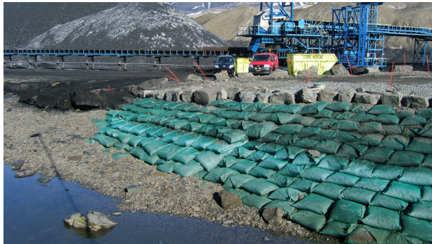
Figure 17. The Kapp Amsterdam quay wall stabilised with the geobags
