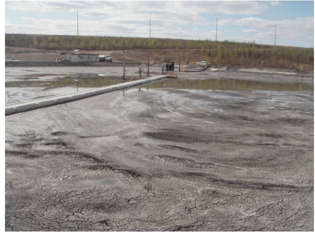
Figure 10. View of MFT deposit surface on April 26, 2010 (eight months after pit filling).
