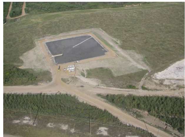
Figure 3. Aerial view of dewatering pit shortly after pit filled.
