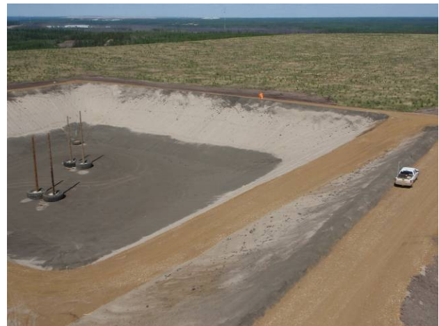
Figure 1. View of containment pit prior to filling.
