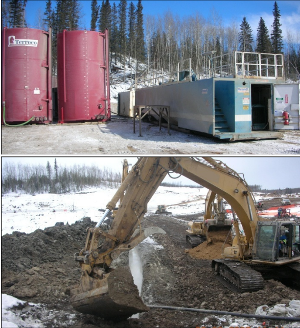
Figure 10. Above: Batch Plant, Lower: Slurry Wall Construction.
