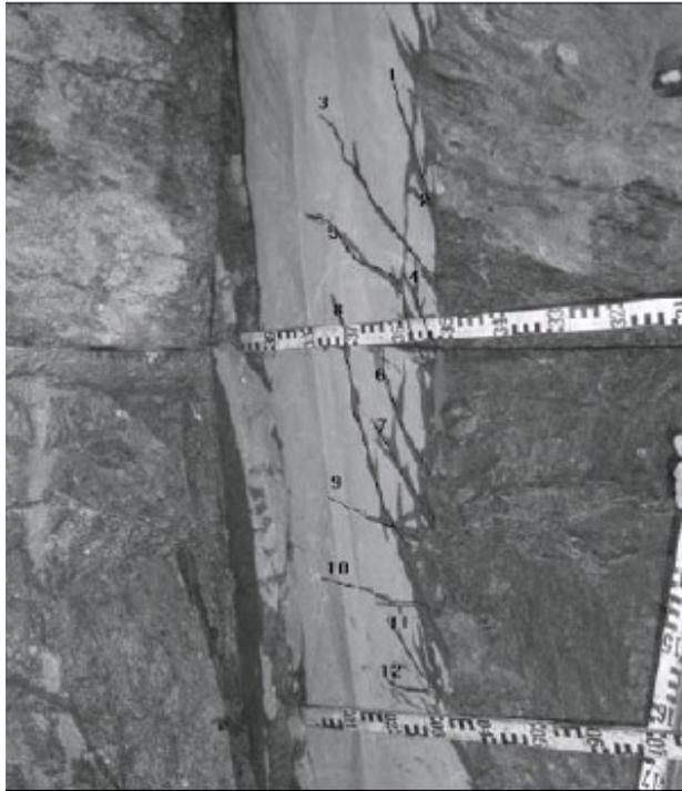
Figure 3: Fractures generated by TBM in cut-away slot at the Aspo HRL, showing upward orientations (Jonsson et al. 2009).
