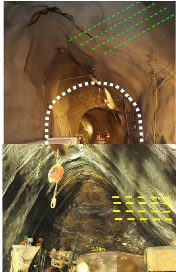
Figure 6: Overbreak pictures from the Mont Terri URL (above) and the Niagara Tunnel Project (below), from Blumling et al. 2007 and Perras 2009 respectively, showing bedding plane orientations.
