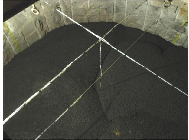
Figure 7. Support cables during the upper concrete pour
