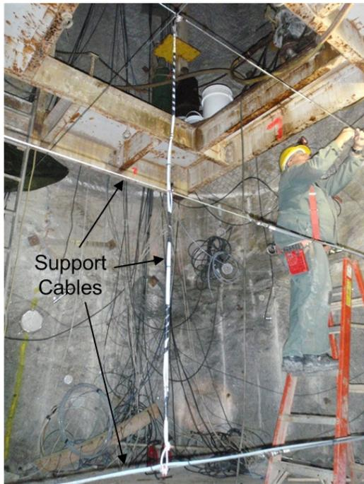
Figure 6. Support cables during instrument installation in the upper concrete component
