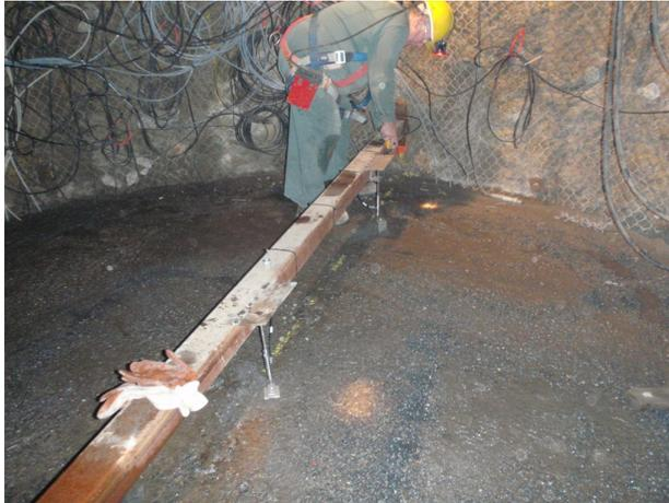
Figure 8. FODT mounting beam above the shaft seal
