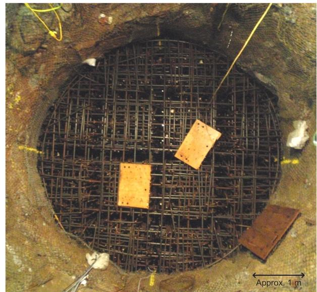
Figure 3. Top view of lower concrete component rebar
