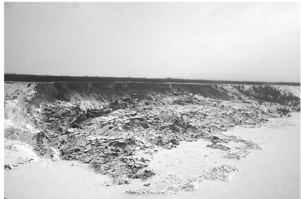
Figure 3. Example of slope failure that occurred in 1997 in frozen glaciolacustrine sediments in the bank of the Mackenzie River, south of Old Fort Point, Northwest Territories. (GSC-ESS Photo 2000-93).
