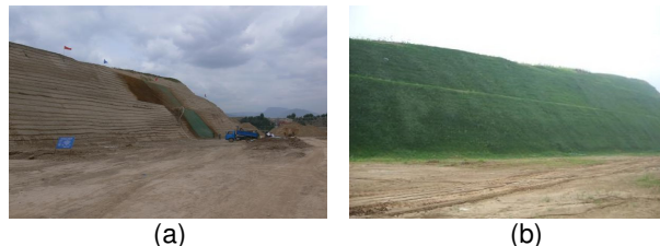
Figure 11. Field application of the slope protection with vegetation along the expressway from Pingliang to Dingxi. (a) slope before protection; and (b) slope after protection
