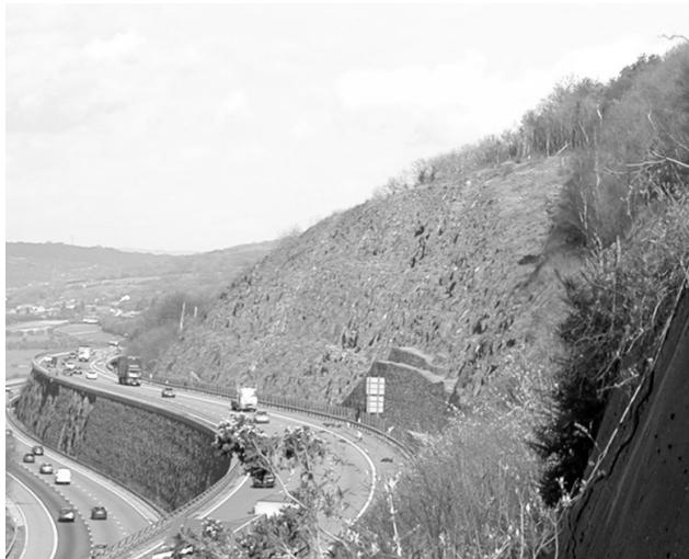
Figure 8. M5 Wynhol Viaduct rock slopes, line of two benches just visible.
