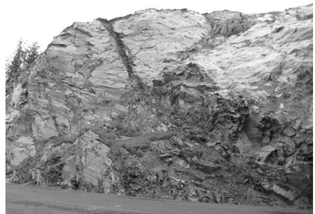
Figure 7. Slope following excavation with large potential wedge/plane failures removed.
