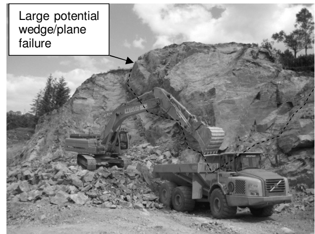
Figure 6. Slope with large potential wedge/plane failure identified during excavation.
