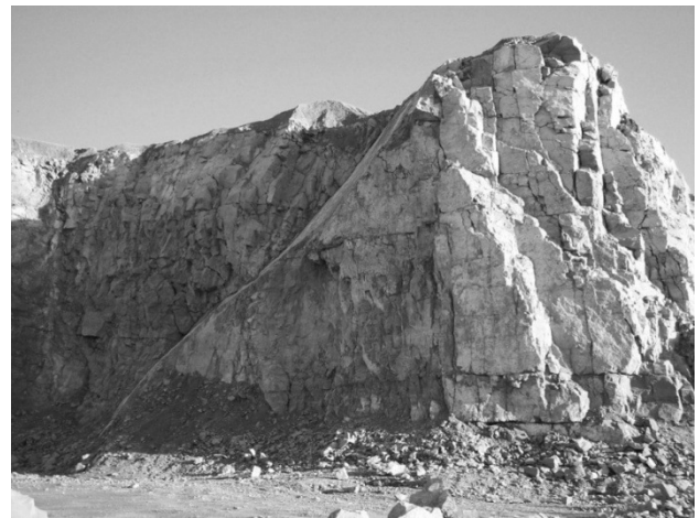
Figure 10. Red Slope (>15m with significant geotechnical features).
