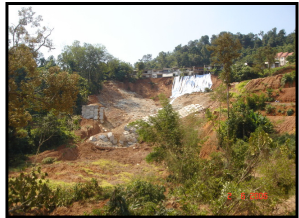
Figure 7. Reinforced soil wall collapsed.
