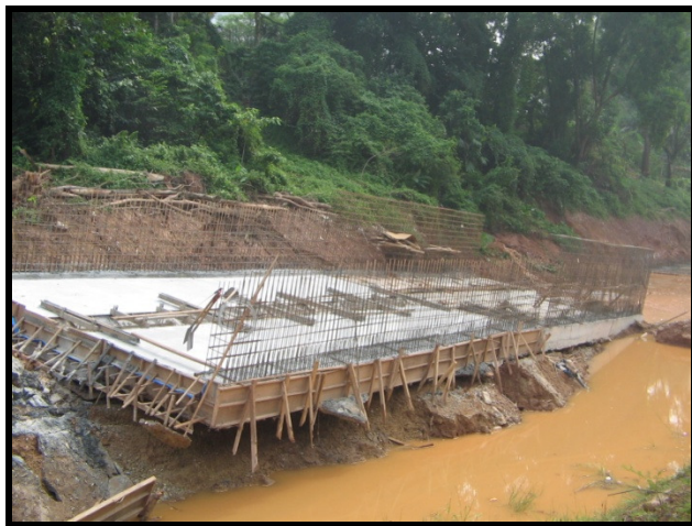
Figure 10. The construction of monsoon drain.
