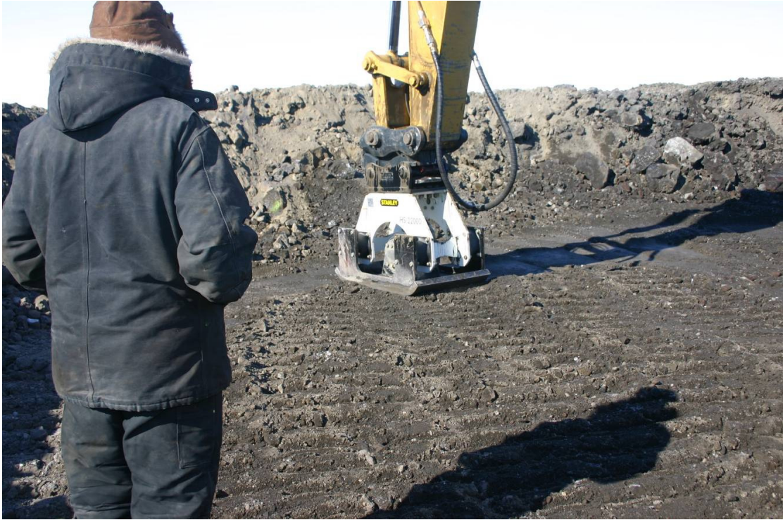
Figure 9. Wind turbine #1; recompaction of excavated fill with large hydraulic plate compactor.
