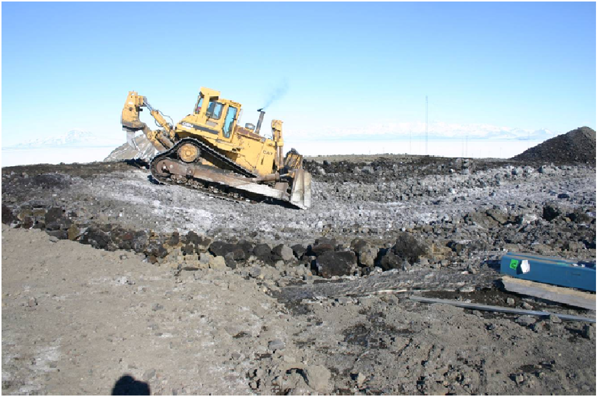
Figure 7. View of excavation of foundation soils, November 2008.
