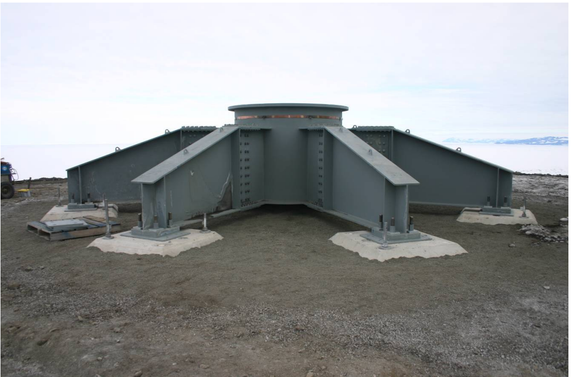
Figure 10. Wind turbine #1; foundation steelwork in place.
