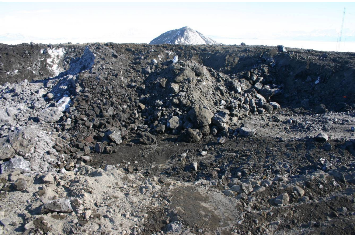
Figure 8. Wind turbine #1 foundation; material near base of excavation.
