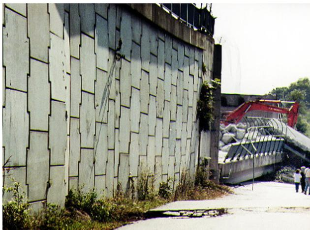
Figure 1. Arifiye Reinforced, earth bridge approach MSE wall (Izmit earthquake, 1999), From SoilTech 2000
