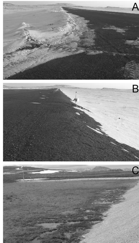
Figure 7. Snow accumulation on the Southeast (A) and Northwest (B) shoulders and toes of the airfield embankment on April 2005. C) Drainage problem at the Northwest toe of the airfield embankment on July 2004 at Tasiujaq Airport, Northern Quebec, Canada. (photographs by Frédéric Vinet, CEN)
