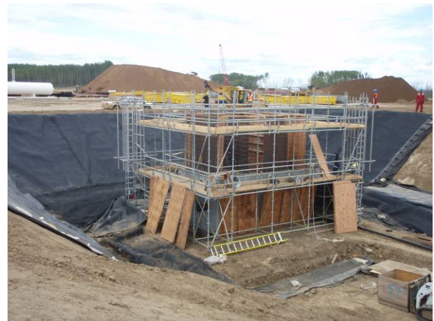
Figure 1: Liner installed under/behind Supernatant Sump. Note backfill protection under concrete structure.
