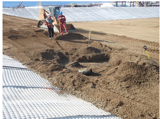
Figure 6: Damage to liner caused by forklift removal of the rig mats.
