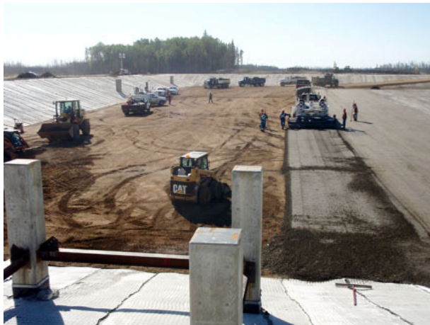
Figure 5: Installation of roller compacted concrete.
