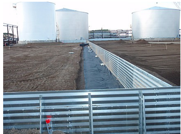
Figure 4: Steel containment berms showing external support posts and liner attachment to the bottom of the berm inside the wall.
