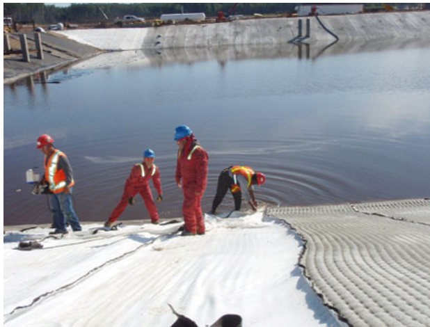
Figure 3: Installation of concrete filled fabric forms. Note that the pond is being water tested during this part of the installation.
