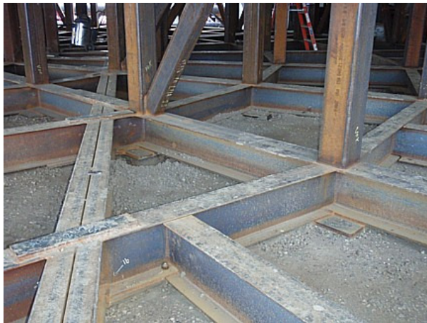
Figure 2: Support structure underneath the warm lime softener tank. With this type of detail only a spray-on liner will be effective.
