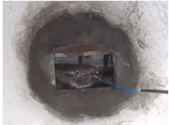
Figure 14. Final opening of the siphon
