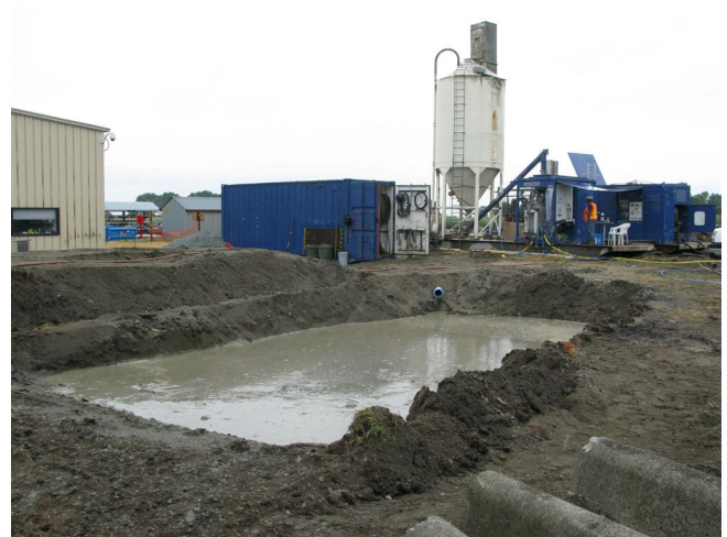
Figure 8. Mud pit and grout plant
