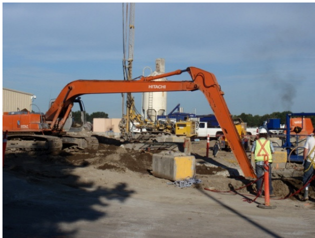
Figure 10. Excavation with long-arm backhoe
