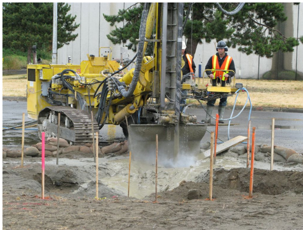
Figure 7. Drill rig excuting chamber wall column
