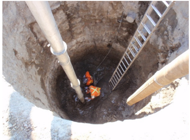
Figure 11. Completion of shaft using vacuum line
