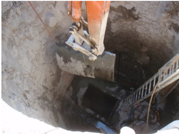
Figure 13. Completed chamber with siphon exposed
