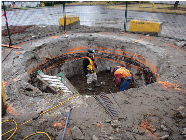
Figure 9. Shoring ring installation in upper shaft
