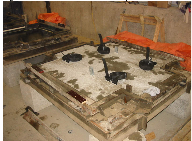
Figure 6. Connection Sleeve and Strip Cast into Panel
