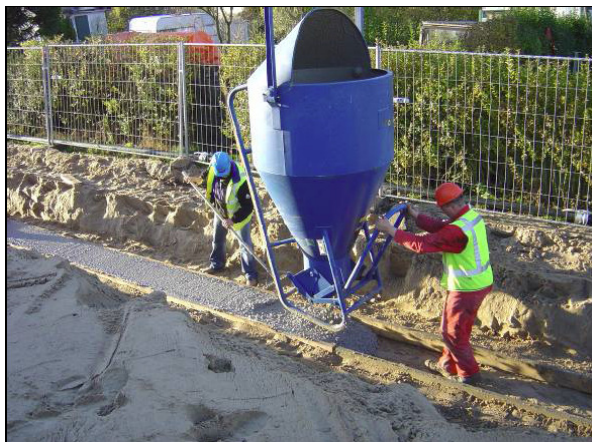
Figure 10. Casting of leveling pad
