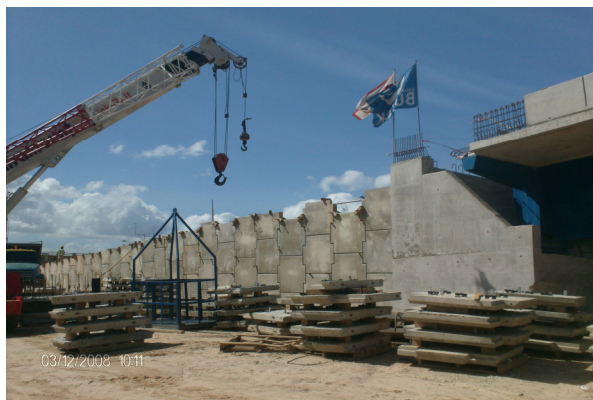
Figure 15. MSE Wall Installation
