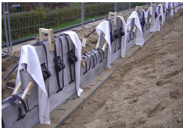
Figure 11. First row of panels sitting on leveling pad
