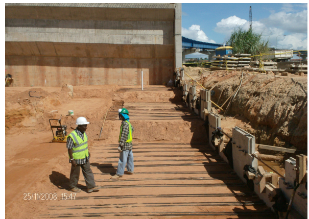
Figure 13. Geosynthetic strips laid flat
