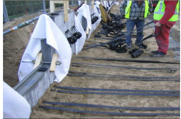
Figure 12. Geosynthetic strips being unrolled on backfill
