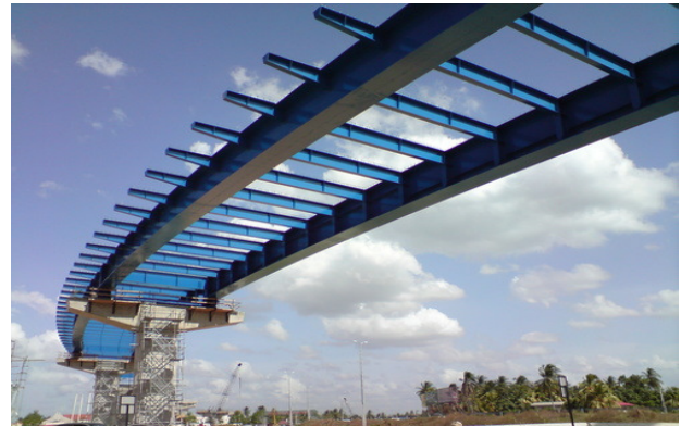
Figure 3. Bridge Superstructure before decking
