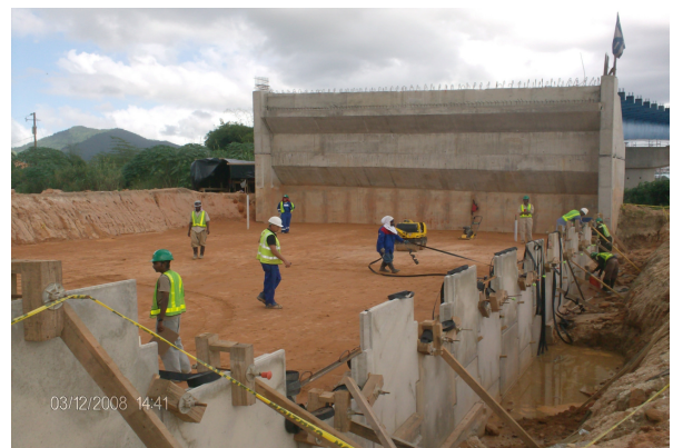
Figure 14. MSE Wall Installation
