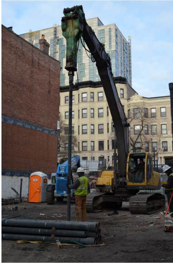
Figure 1. Picture of Ductile Iron Pile Installation
