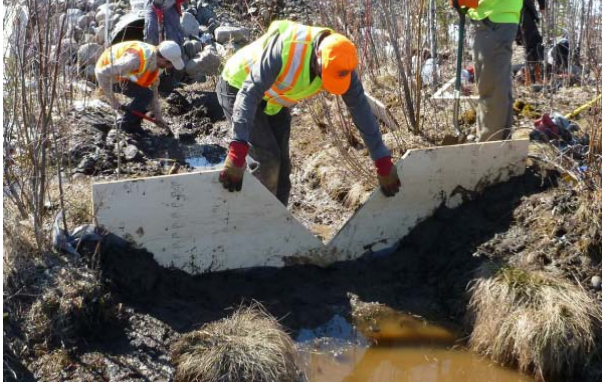
Figure 3 : V notch weir at Beaver Creek site
