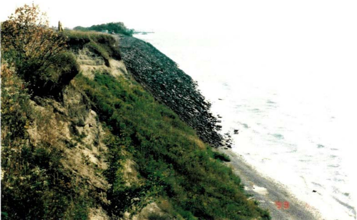
Figure 8. Completed Dynamic Revetment
