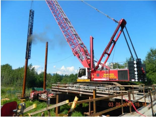
Figure 8. Pile driving crane and hammer.
