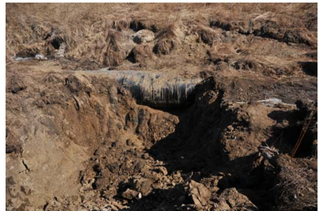
Figure 5. Thermal insulation of the CRCOP near Amuer, northern Heilongjiang Province, China (photographed on April 15, 2012)
