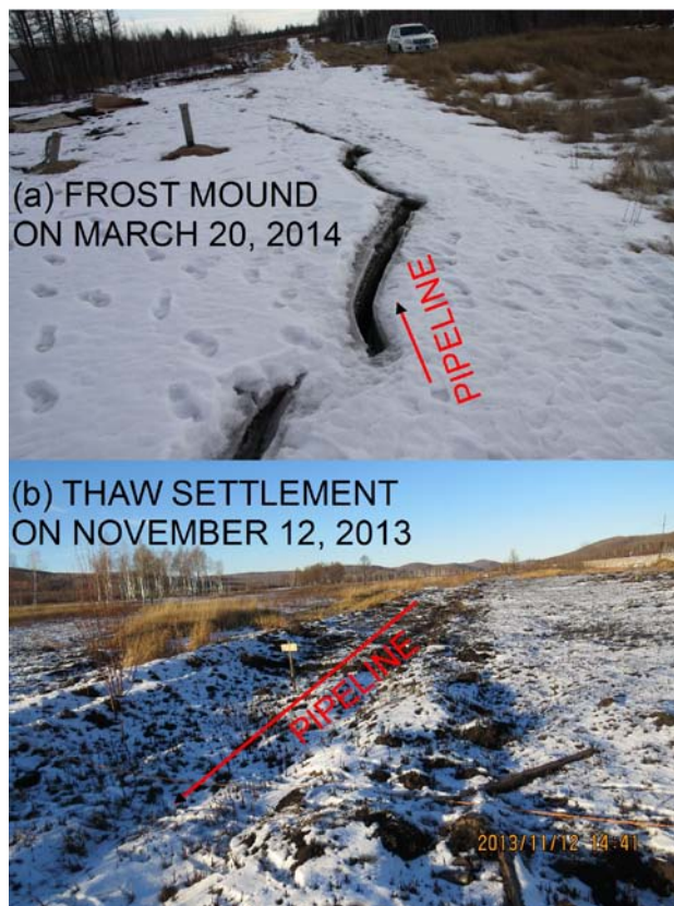
Figure 2. The example of frost hazards along the CRCOP
