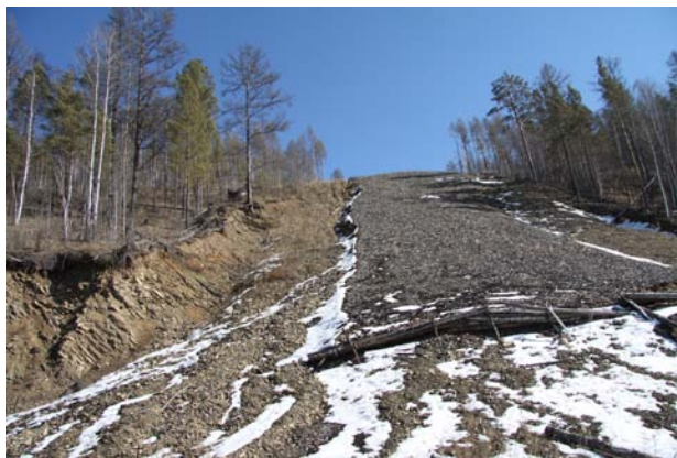
Figure 3. Woodchip layers of a slope surface insulation along the CRCOP on March 23, 2014
