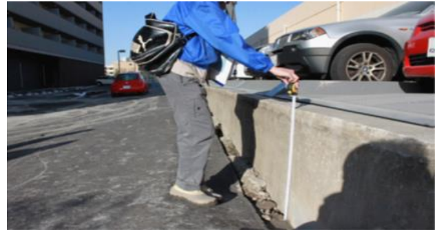
Fig. 2. Uplift of underground parking lot (Tokimatsua et al. 2012).
