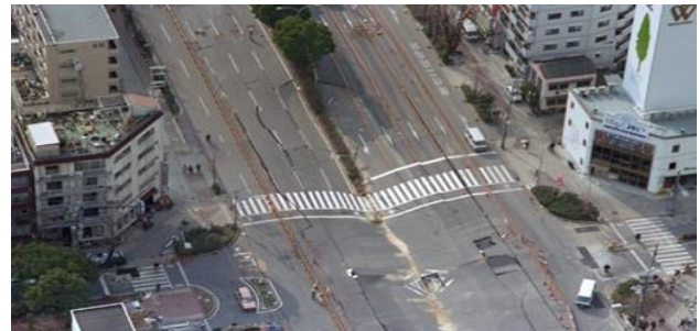
Fig. 3. Daikai Station failure - Niigata-Chuetsu Earthquake ( http://kobe117shinsai.jp/area/hyogo/d037.php )
