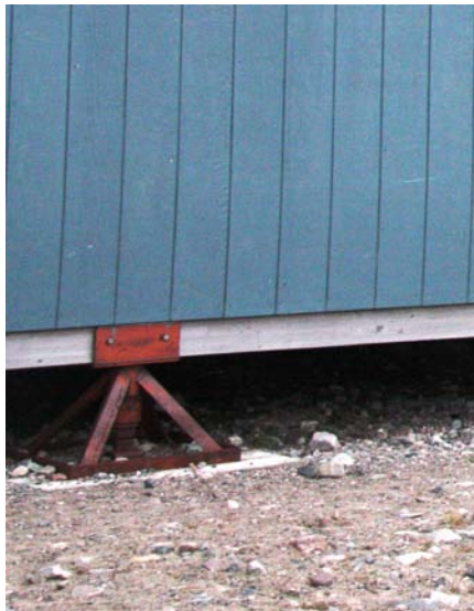
Figure 2. Screw jacks being used in Arviat, Nunavut
