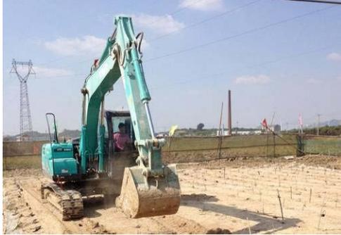
Figure 8 Picture showing the excavator can run on the ground surface after EO
