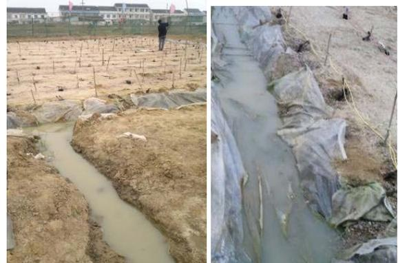
Figure 5. Picture showing the drained water in the drainage ditch using the high power supply of 80V/2000A
