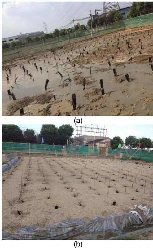
Figure 3. Pictures showing the ECWD installation in the field: (a) After completing the ECWD installation; (b) After placing the sand mat and the connection of electric wires.
