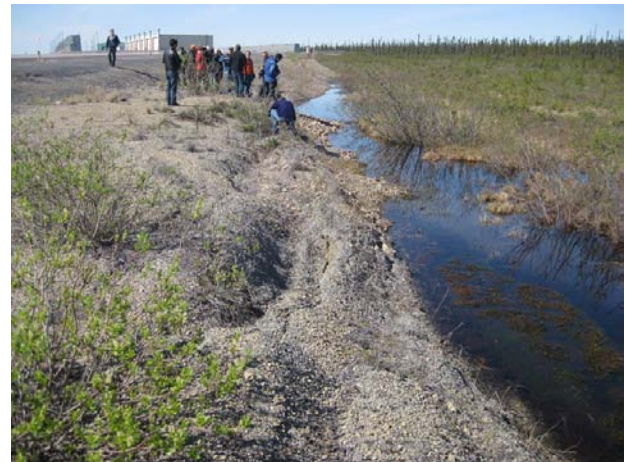
Figure 7. Runoff collecting along east side of Taxiway E, and associated subsidence; summer 2011
