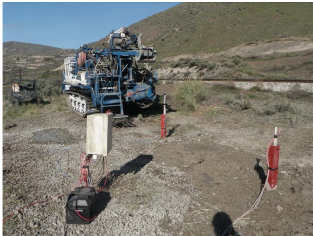
Figure 4: Piezometer and Shape Accel Array installation at the Ripley Landslide in April 2013.
