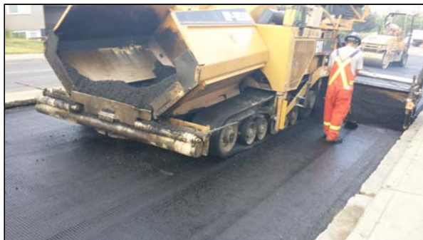
Figure 5. Fiberglass grid installed over the first lift of asphalt concrete.
