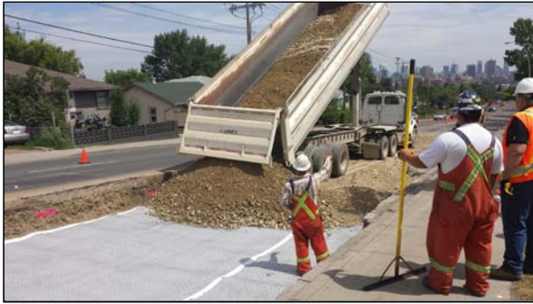
Figure 3. Laying of biaxial geogrid composite
