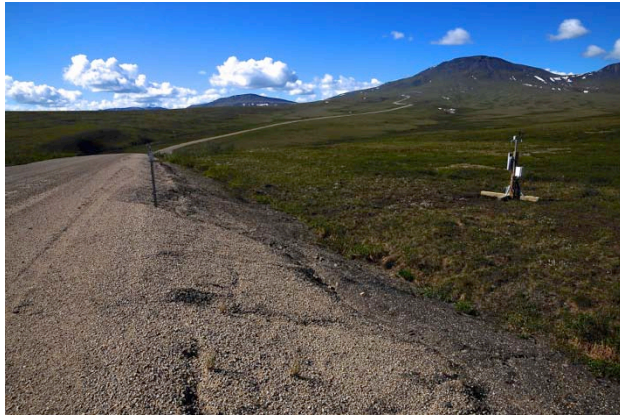
Figure 4. Long-term embankment instability over shallow ice wedges, Dempster Highway, NT-km 8.5, June 2015 photo
