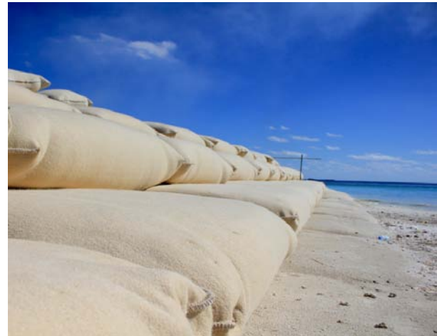
Figure 3 Typical GSC coastal protection revetments
