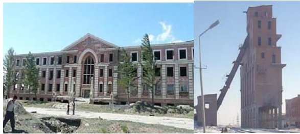
Figure 4. Administrative building (above) and entrance of vertical shaft of Nalaikh coal mining plant with ventilation hollow
