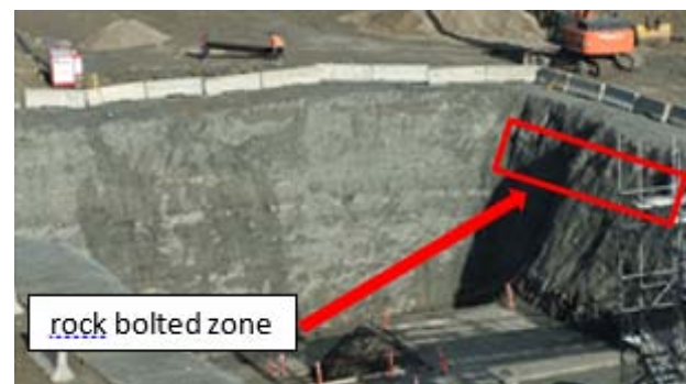
Figure 5: Example of Rock Bolted Zone
