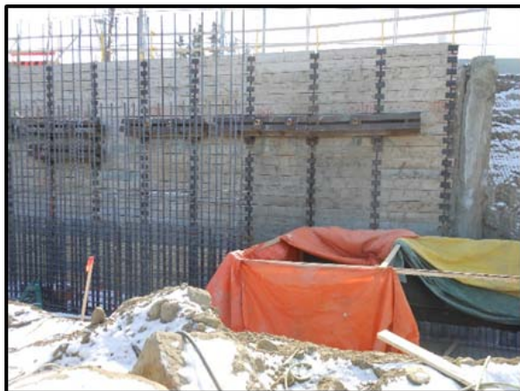
Figure 1D - 0.5H:1V globally stable slopes offer reduced excavated volumes relative to Figure 1A with modest slope protection
