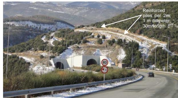
Fig. 4. Support Measures for S3 Tunnel; (a) figure of support measures implemented (modified after Koronakis et al., 2004) and, (b) Photo of reinforced slope/twin tunnel portals.
