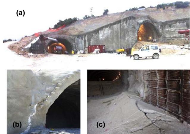
Fig. 3. Photos from S3 Tunnel Construction; (a) Eastern Portals; (b) cracks within shotcrete adjacent to tunnel walls; (c) upheaval of invert.
