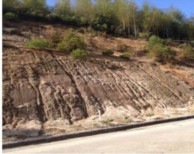
Fig.1 A typical slope failure due to freeze-thaw cycles in Fujian province
