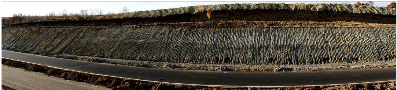
Figure 3. The cutting slope after excavated (2010.09)
