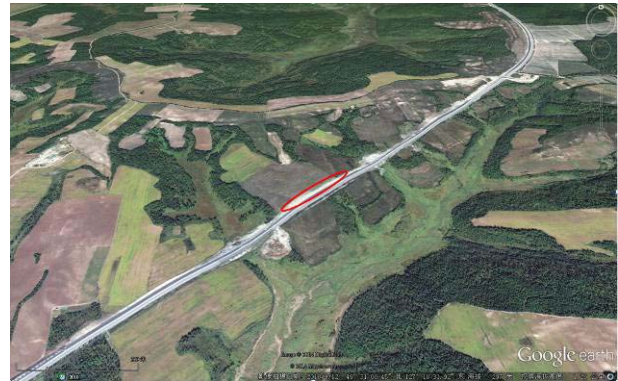
Figure 2. The Location of cutting slope (photo from Google earth)
