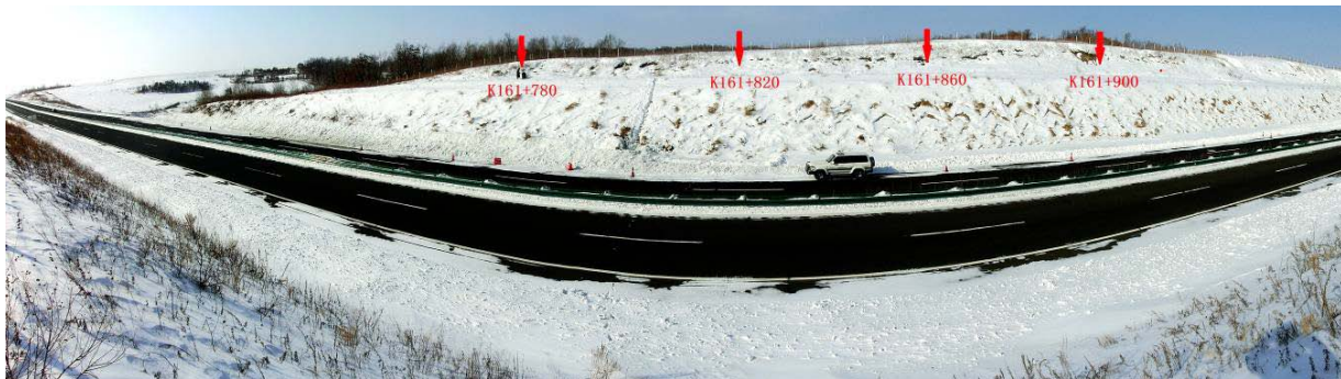
Figure 7. The position of monitoring borehole on left slope of K161 + 640-K162 + 200 section
