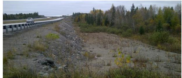
Figure 2. Photograph of the 10 m high SBL embankment looking south from north limits.
