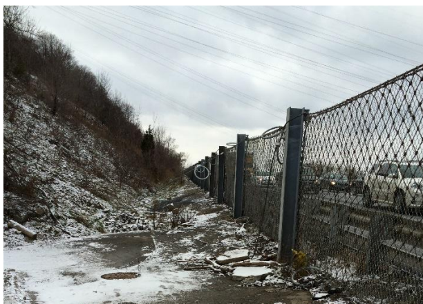
Figure 2. Typical site conditions at highway level, showing the talus slope, ditch, catchment fence, and travelled lanes.
