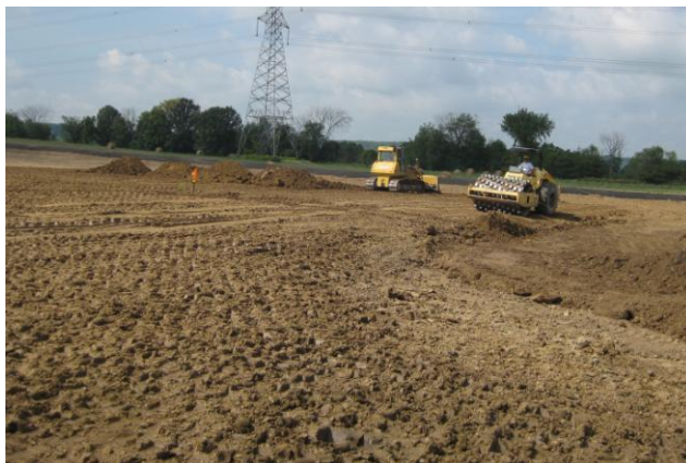
Figure 3b. Compaction Activity of Project DV
