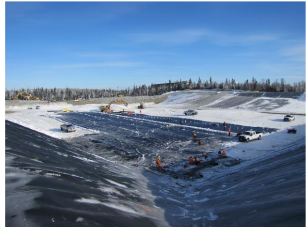
Figure 7. General view of tailing pond during construction
