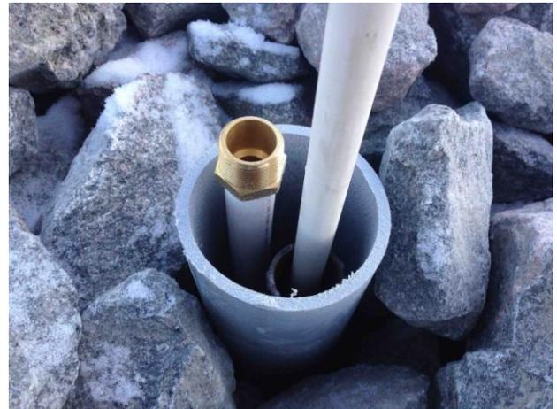
Figure 9. The tremie tube has been inserted in the steel pipe. The PEX pipe to contain the thermistor string is seen alongside. A larger PVC pipe protects the system.
