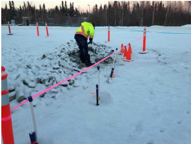
Figure 6. All convection pipes and thermistor string holders have been placed to a depth of 6 m below the original ground surface. ACE construction begins.
