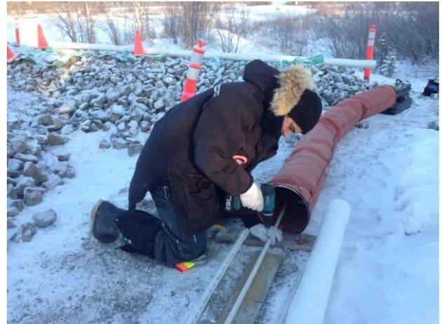
Figure 8. Holes are drilled in the bottom of the tremie tube (described in section 4.2) to facilitate the second airway.
