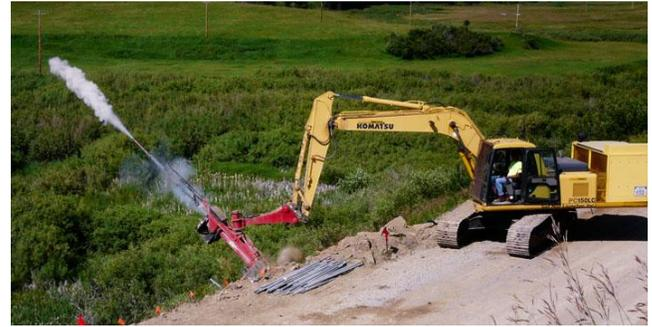
Figure 3. A compressed air launcher (GSI, 2015) greatly increases the installation speed of the CPC pipes over conventional drill and install methods.
