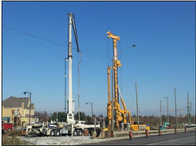
Figure 3.1 - Bauer BG36H & modified 42m (boom length) concrete pump with a 20m long tremie hose attached
