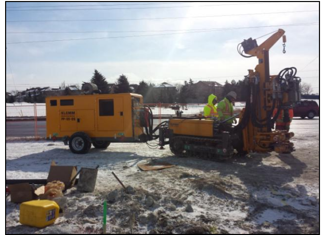
Figure 5.3 - Klemm 702-2 vertical drill used for remedial grouting
