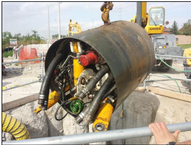
Figure 5.5 Split TBM being removed from R1 (cutting wheel facing away from photograph)
