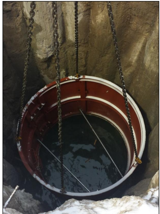
Figure 5.1 Lowering a steel circular form to sit on the tremie plug – concrete poured on outside of steel form
