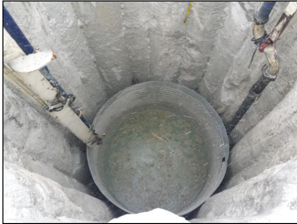
Figure 5.2 - 3.3m diameter corrugated steel culvert pipe used to reline shafts
