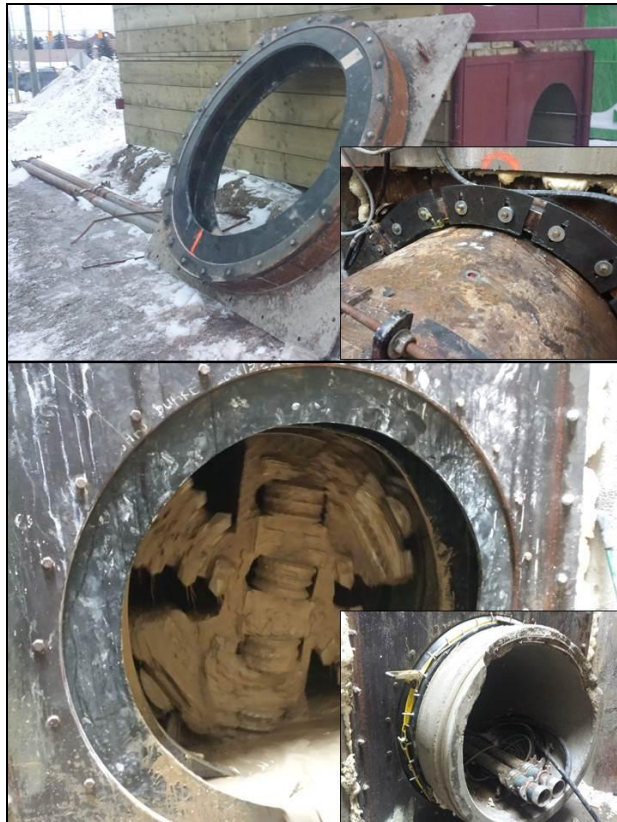
Figure 5.4 Tunnelling launch (top) and reception (bottom) seals
