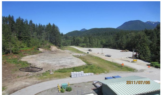
Photograph 2. View of pre-development site looking north. Chlorination building in foreground.
