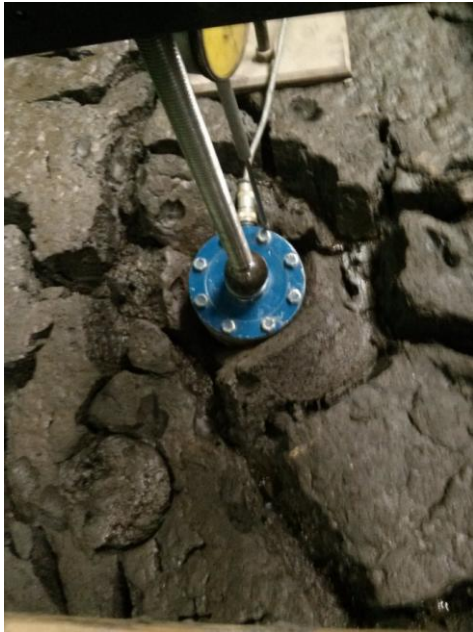
Figure 9 “Punching Shear” failure mechanism after the 70% SC bearing capacity test
