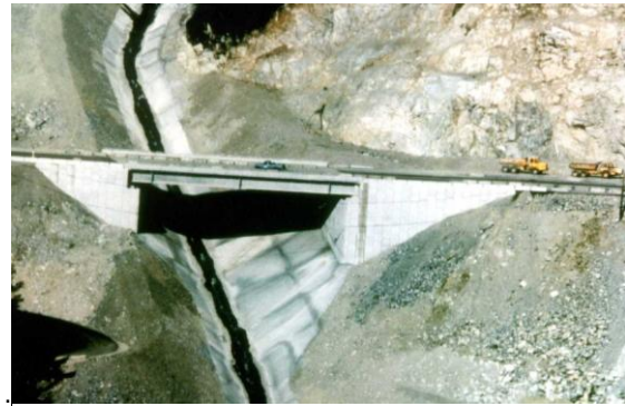
Figure 5. Debris Channel – Fraser Creek, B.C.
