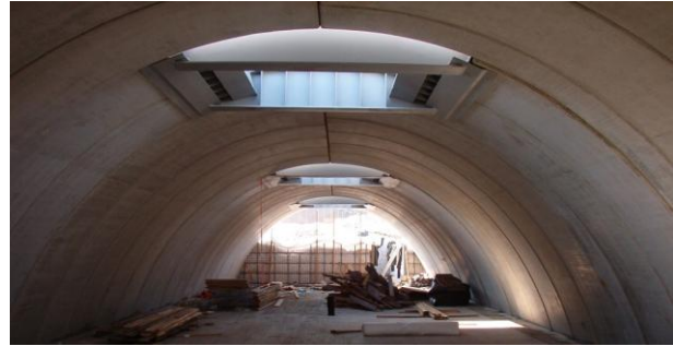
Figure 4. Top Windows in a concrete culvert
