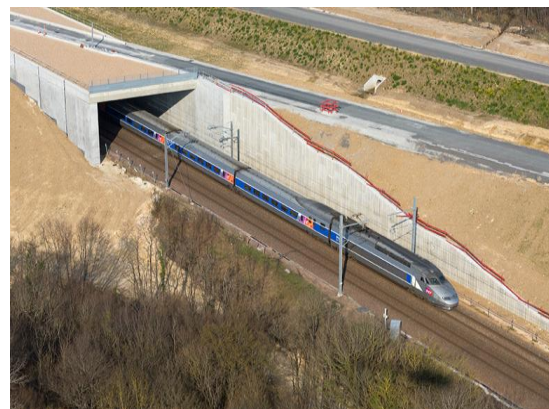
Figure 1. An MSE wall alongside a railway
