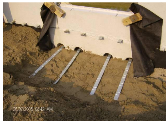
Figure 12. Test strip placement at/behind a test panel
